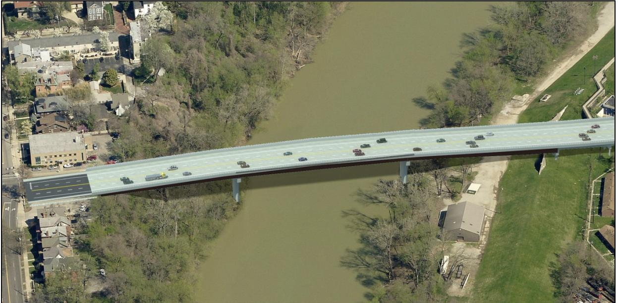
Figure 25: Steel Plate Girder Alternative Layout
